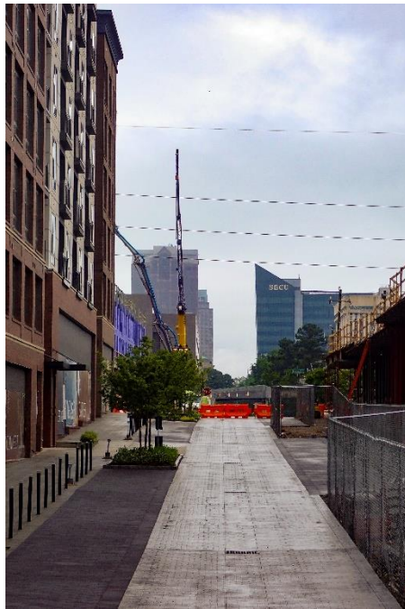
Figure 3 - Seaboard Station (April 2023)
